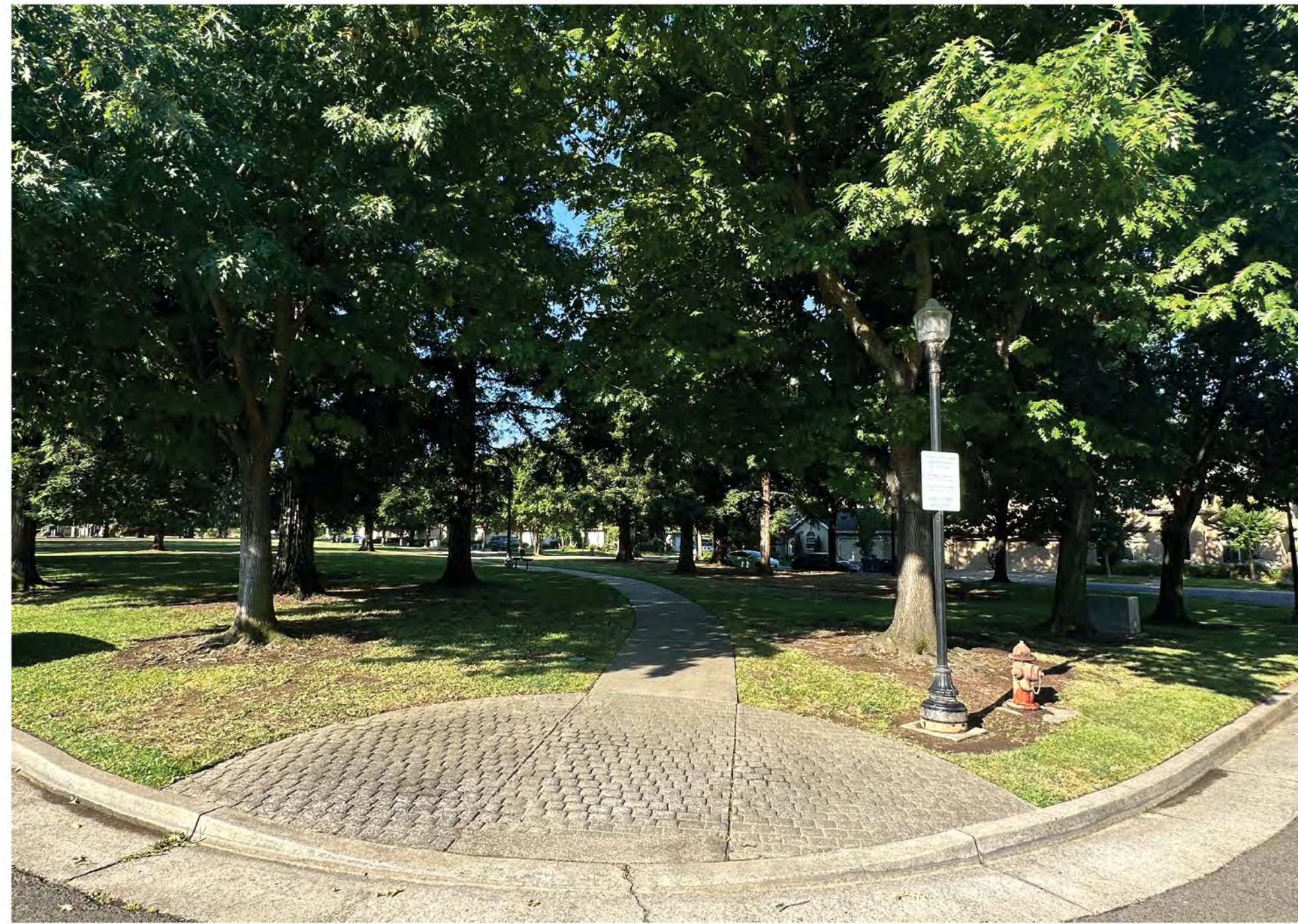
View of North Access Ramp
