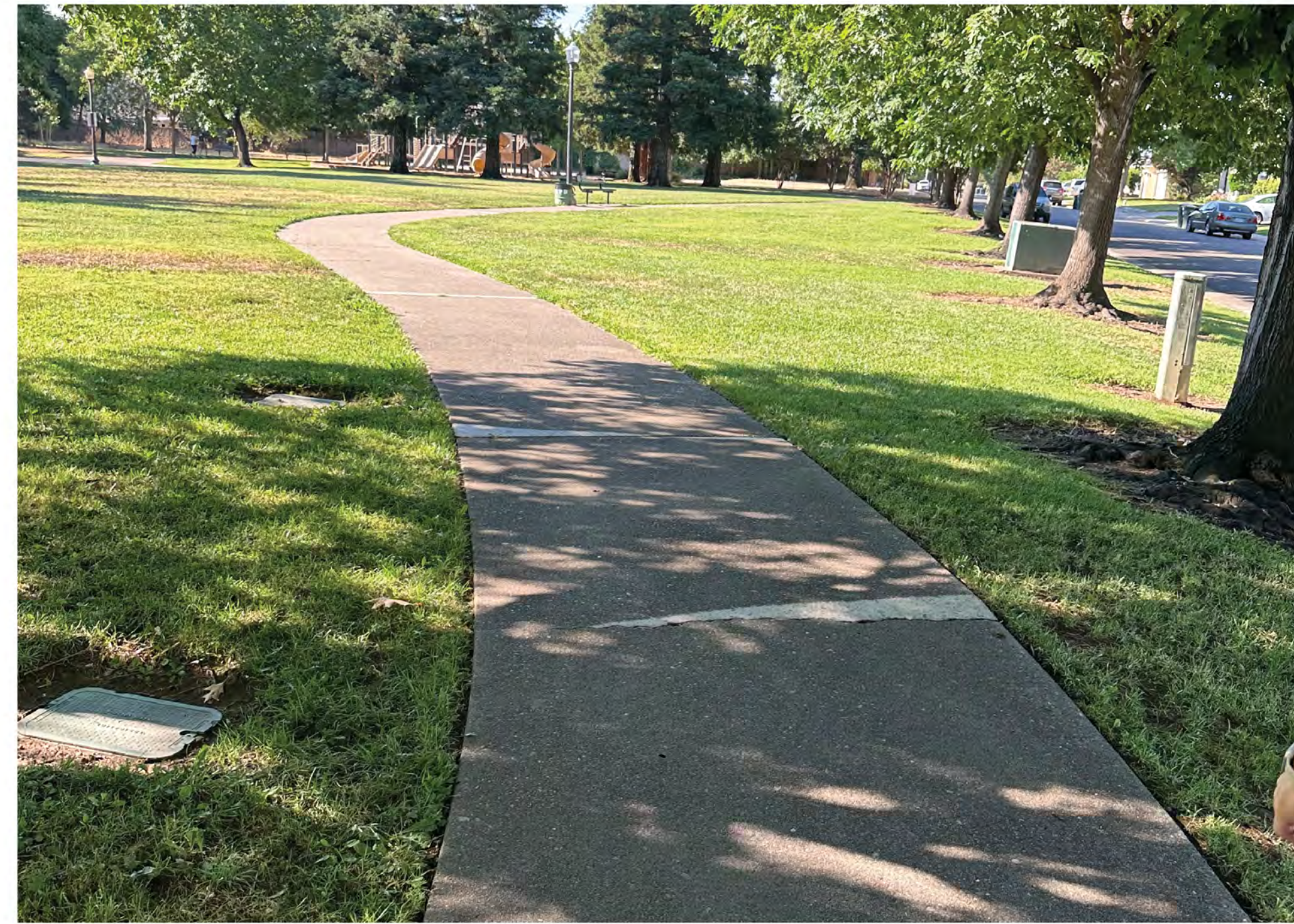
View of Concrete pathway looking South
